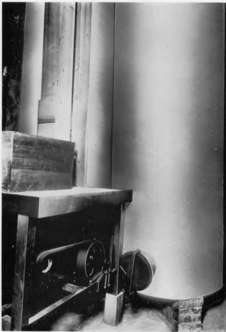
Photo. 1. Concrete silos specially constructed for the storage experiment of rice.
